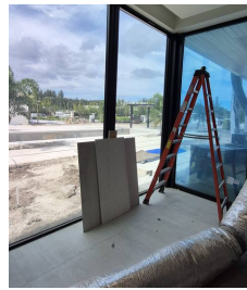
Ducts and lumber in front of the glass
