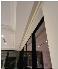
Glydea tracks fitted in the pockets
